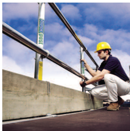
N.B. Handrail posts are required every 1.5m.
